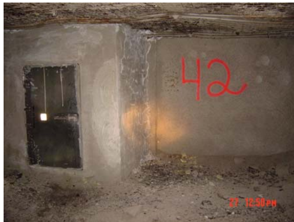
Concrete Block Stopping in Excellent Condition.
