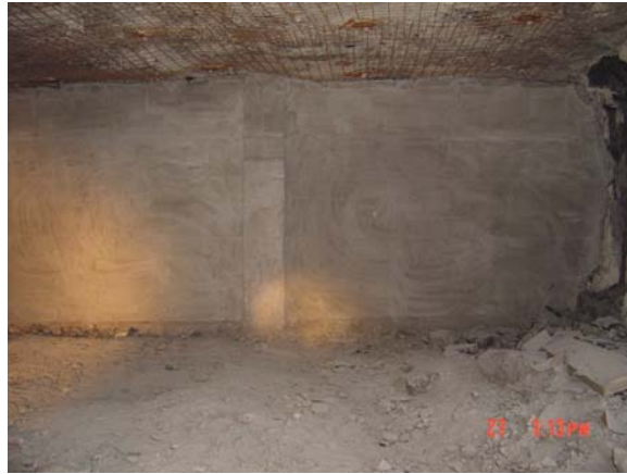
Concrete Block Stopping in Good Condition.
