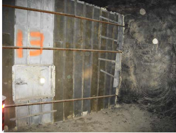
Kennedy Stopping in Good Condition.
