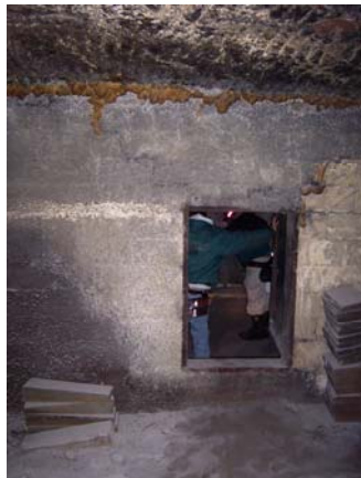
Concrete Block Stopping in Average Condition.
