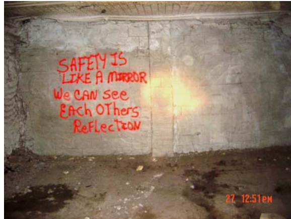
Concrete Block Stopping in Average Condition.
