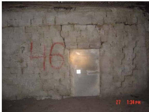
Concrete Block Stopping in Average to Poor Condition.
